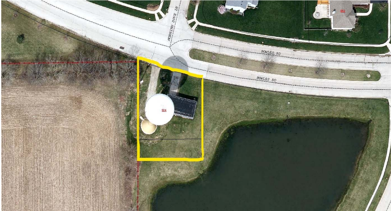
Bowels Road Water Tower Site 924 Bowels Rd., Antioch, IL 60002
