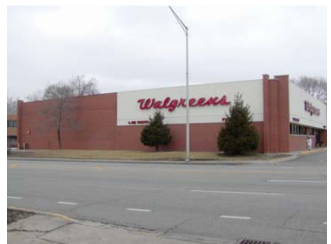
Inadequate fenestration does not allow views into interior spaces.
