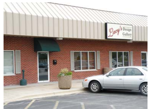
Unattractive/disproportional retail storefront facade character.
