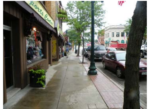
Typical pedestrian "Main Street" streetscape character.
