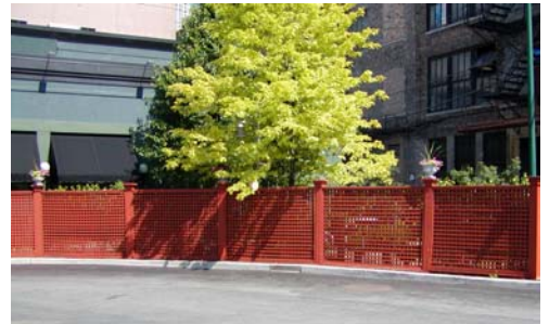
Solid utility screening must be provided.
