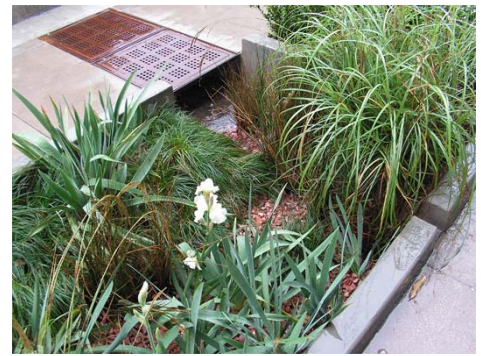
Stormwater filtration through a naturalized bioswale management program.
