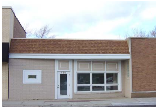
Example of unacceptable retail storefront building facade articulation.
