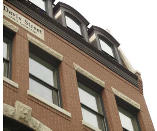
Well-articulated and proportional upper floor fenestration.
