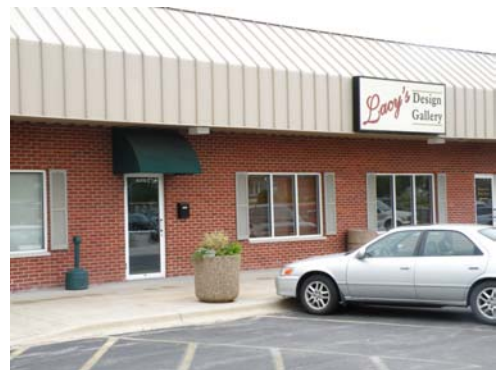
Unattractive/ disproportionate retail storefront facade character.
