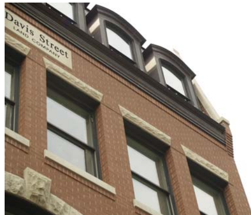
Well-articulated and proportional upper floor fenestration.
