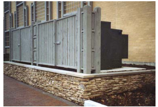
Solid wood fencing is an appropriate material for screening trash or service areas.
