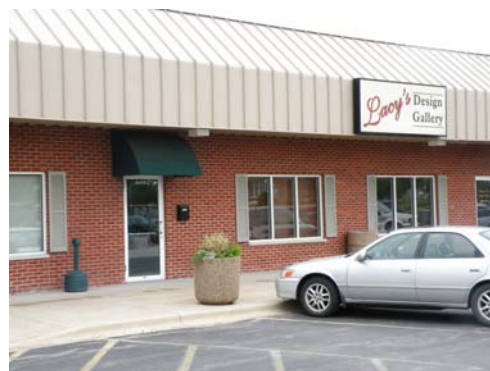
Unattractive / disproportional retail storefront facade character.
